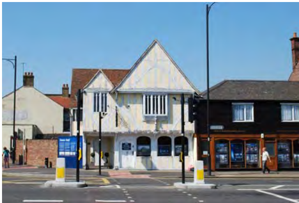
Swan Hall, Victoria Avenue (Victoria Gateway Neighbourhood Policy Area)
