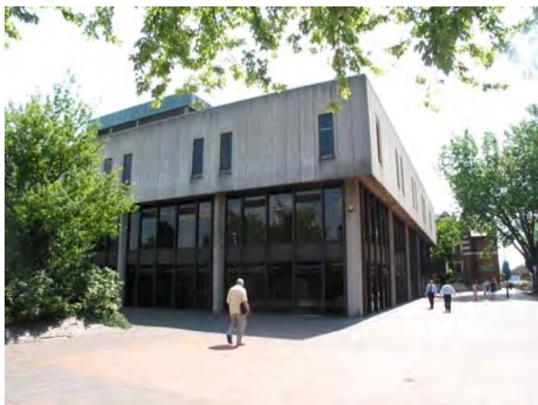
Central Library (former), Victoria Avenue (Victoria Gateway Neighbourhood Policy Area)
